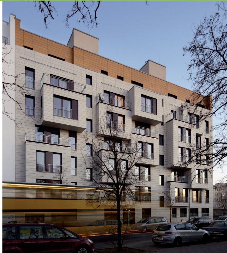
Residential building in Berlin © Architekten Deimel Oelschläger
