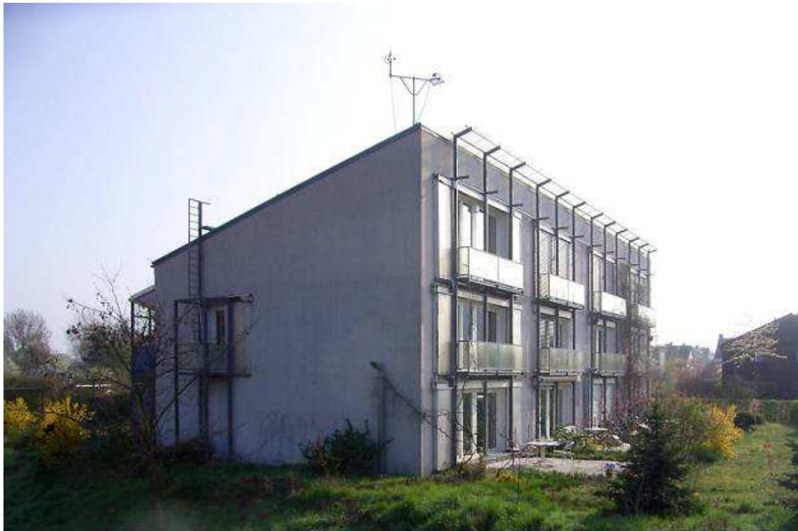
West side of the Passive House in Darmstadt Kranichstein with a small balcony and access ladder to the roof. The weather station is clearly visible. (Photograph: Feist)
