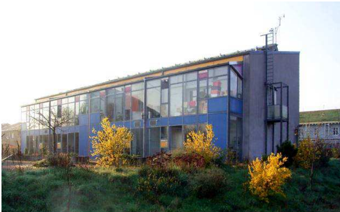
Picture of the Passive House in Darmstadt Kranichstein from the northeast side ; the conservatory can be clearly seen, the air intake grilles of the four separate ventilation systems are visible at the ground floor ceiling level.
