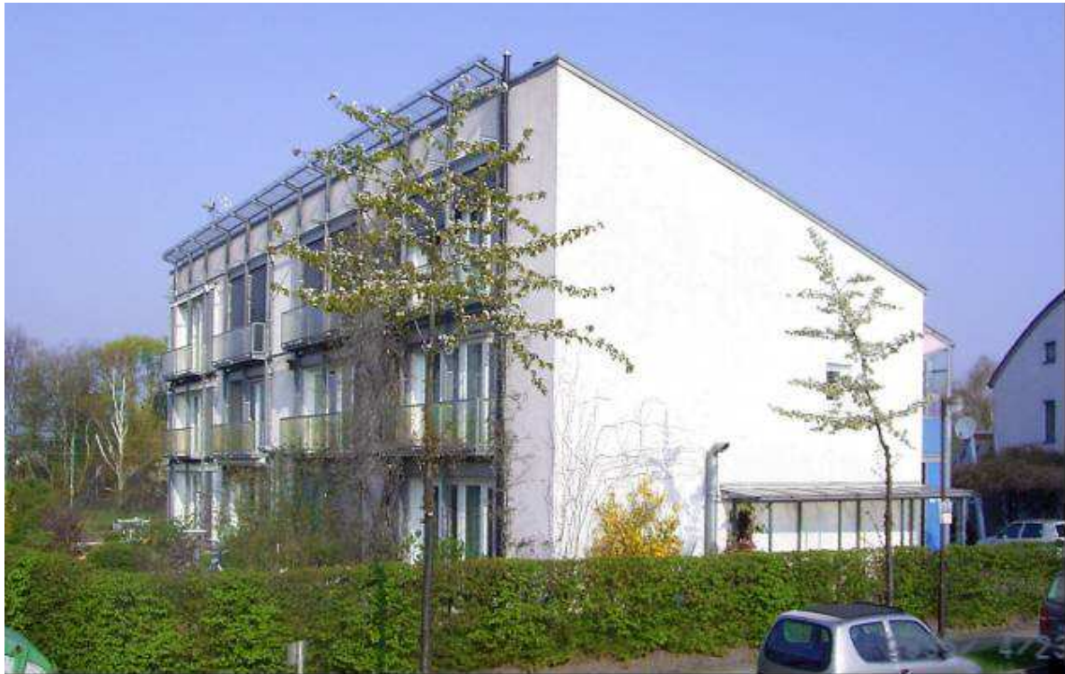
Passive House in Darmstadt Kranichstein, view from the southeast : In the gable wall facing the street, there is only a small east-facing window on the ground floor. The exhaust air outlet and the covered central entrance to the shared basement is clearly visible.
