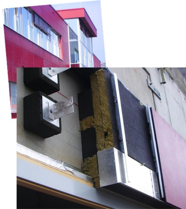
Punctiform thermal bridge: X = 0.02 \dots 0.04 \text{ W/K}
