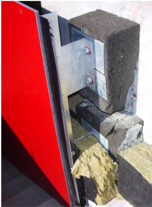
Punctiform thermal bridge: X = 0.02 \dots 0.04 \text{ W/K}
